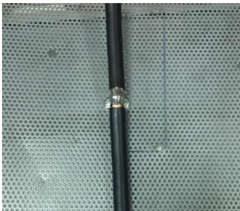
Figure 2: U-shaped metal pipe clamp
